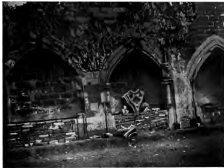
RECESSES OF N. CLOISTER
